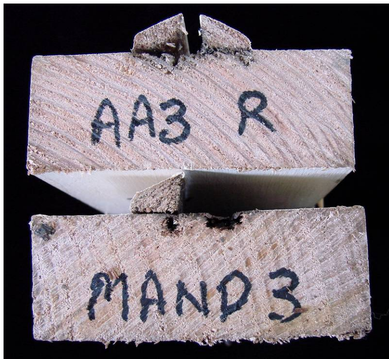
Figure 17. Centre of timber sections cut for inspection, showing 5-6 mm decay and staining under glass edge (removed) and quad beading.
